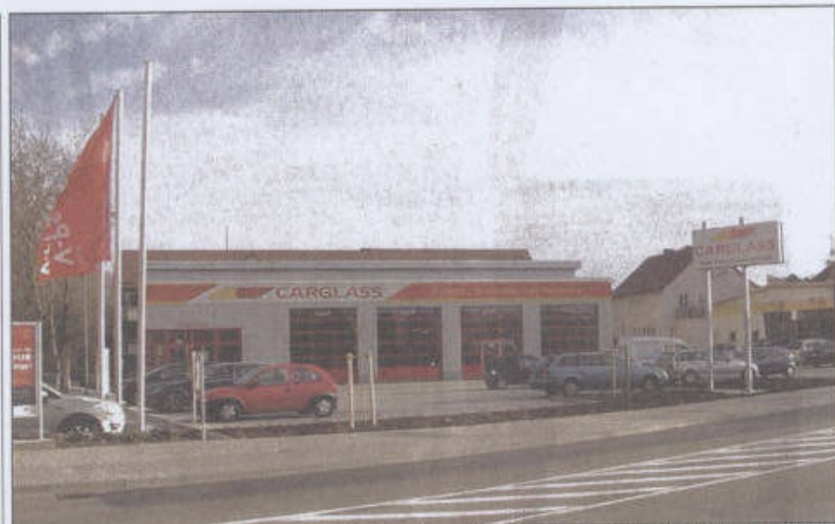
Greenman Investments has let some of its existing auto service centres in Germany to the repair firm Carglass
